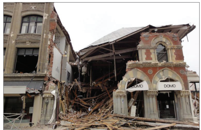
Collapse of URM building - 2011 M_w 6.1 Christchurch, New Zealand earthquake. Photo: EERI/Justin Marshall.
