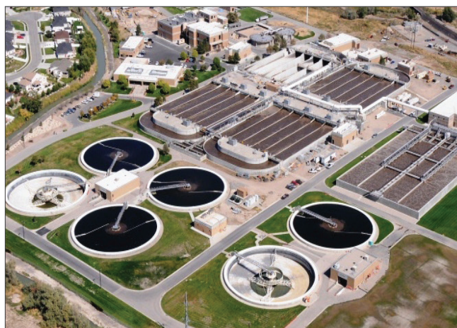
Wastewater treatment plant located in Salt Lake County. Photo courtesy of South Valley Water Reclamation
