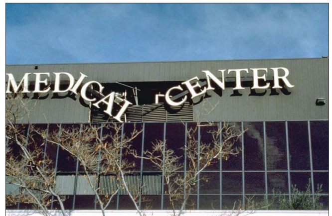
HVAC service outage at the Holy Cross Medical Center in Sylmar caused evacuation of all patients. The damage shown occurred when suspended fans in the penthouse swung and impacted louver panels. This building, a steel frame, also suffered many weld fractures that were not discovered until well after the facility had been restored to service - 1994 M_w 6.7 Northridge, California earthquake. Photo: EERI.
