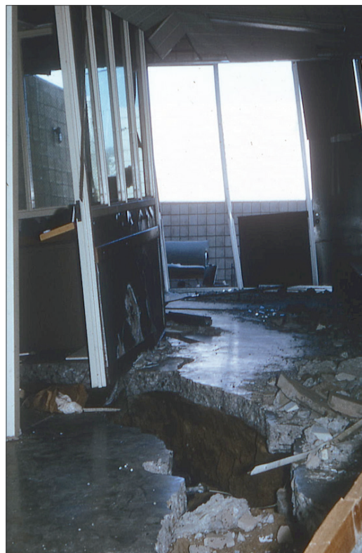
Figure 13. View of interior of building pulled apart by liquefaction-induced lateral spread at San Fernando Juvenile Hall during the 1971 San Fernando, California earthquake. Photo by T.L. Youd.
