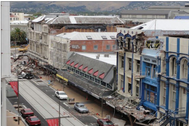
Damage to Central Business District. Mostly collapse of URM - 2011 M_w 6.1 Christchurch, New Zealand earthquake. Photo: EERI/Mary Comerio.
