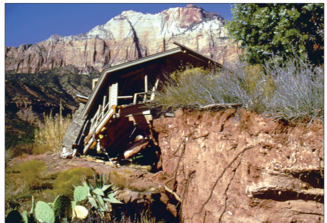
Figure 24. Damage to a home caused by the Springdale landslide in the 1992 M 5.8 St. George earthquake.
