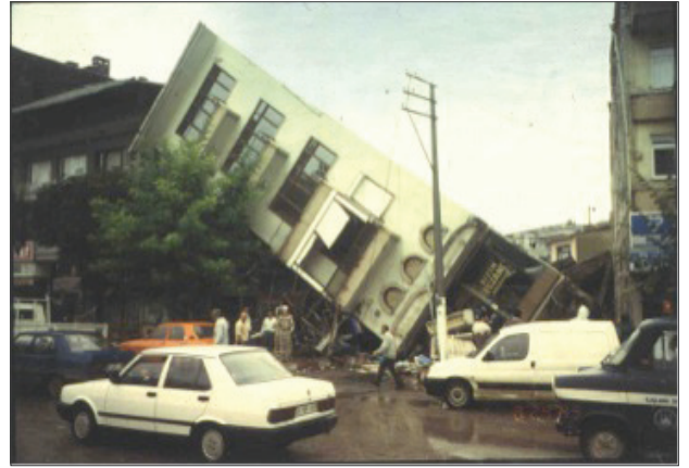
Figure 17. Building in Adapazari, Turkey that tipped over due loss of bearing capacity during the 1999 Kocaeli, Turkey earthquake. Photo by T.L. Youd.
