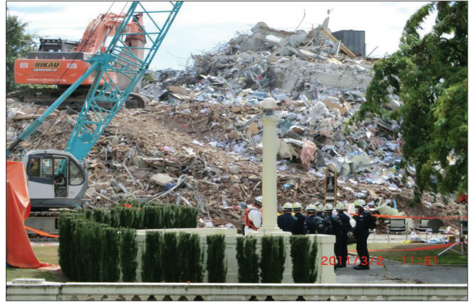
Debris from the catastrophic collapse of the Pyne Gould Corporation - 2011 M_w 6.1 Christchurch, New Zealand earthquake. Photo: EERI/Troy Morgan.
