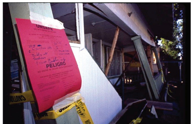
Detail of unsafe posted single family dwelling unit - 1994 M_w 6.7 Northridge, California earthquake. Photo: EERI
