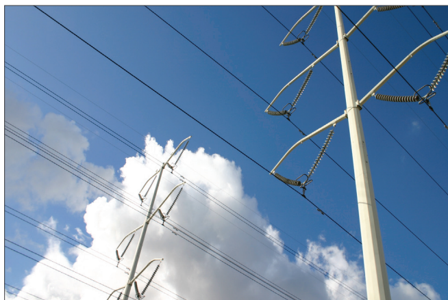
High-voltage electrical transmission lines. Photo courtesy of Rocky Mountain Power.
