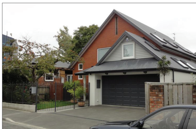
Engineered residential home with extensive foundation with piles. Other homes around the neighborhood suffered significant damage due to liquefaction - 2011 Mw 6.1 Christchurch, New Zealand earthquake. Photo: EERI/Justin Marshall.
