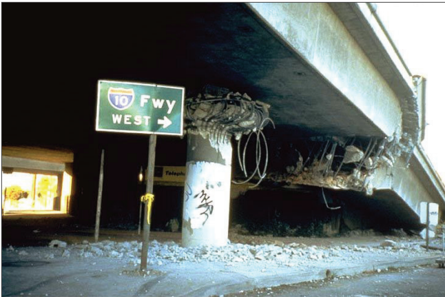
These non-ductile columns failed in shear and then collapsed under the weight of the bridge - 1994 M_w 6.7 Northridge, California earthquake. Photo: EERI.
