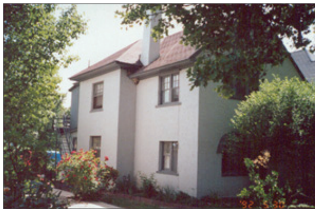
Example two-story URM residence. Photo courtesy of Barry Welliver.
