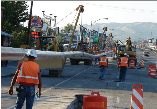
Installation of a welded steel natural gas pipeline in Salt Lake County. Photo courtesy of Quester Gas Company.
