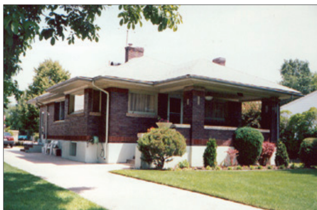
Example one-story URM residence. Photo courtesy of Barry Welliver.
