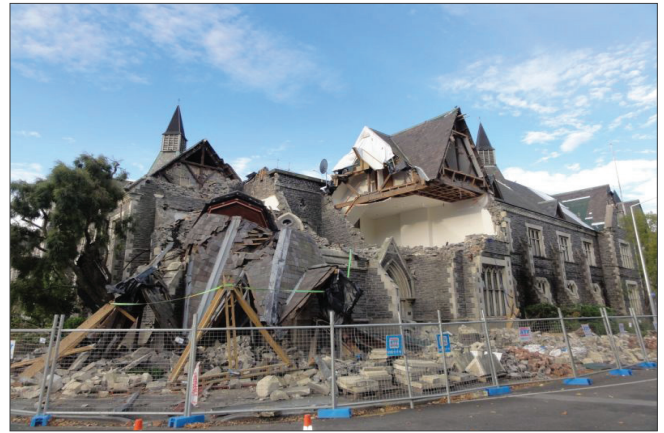
Collapse of URM church - 2011 M_w 6.1 Christchurch, New Zealand earthquake. Photo: EERI/Justin Marshall.
